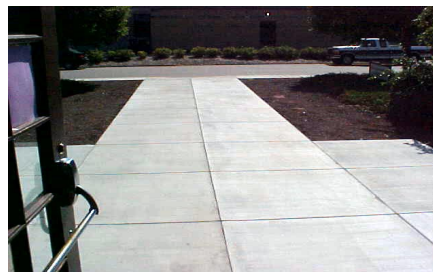
E.C. Activities building (6,047 lbs. of glass)
